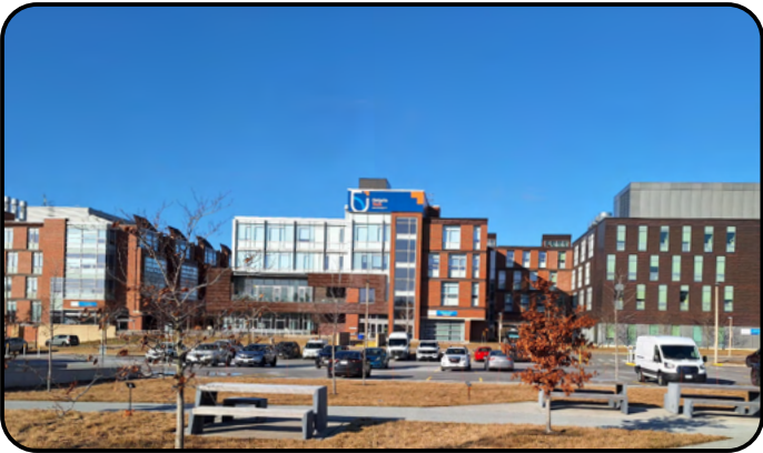
Buildings facing onto Founders Drive
