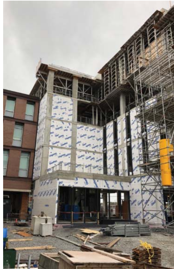
South View – Exterior Sheathing installation
