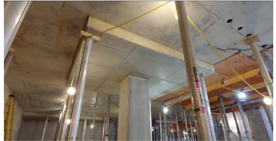
Underside of completed section of Level 1 showing formwork stripped and temporary shoring in place. Column capital also in view.
