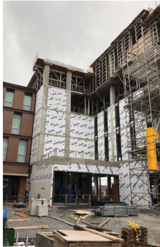
South View – Exterior Sheathing installation
