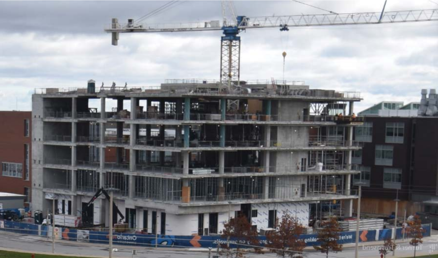
Photo taken 31 October 2020 Northeast elevation
