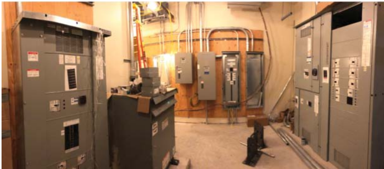
←Electrical Room at LL
