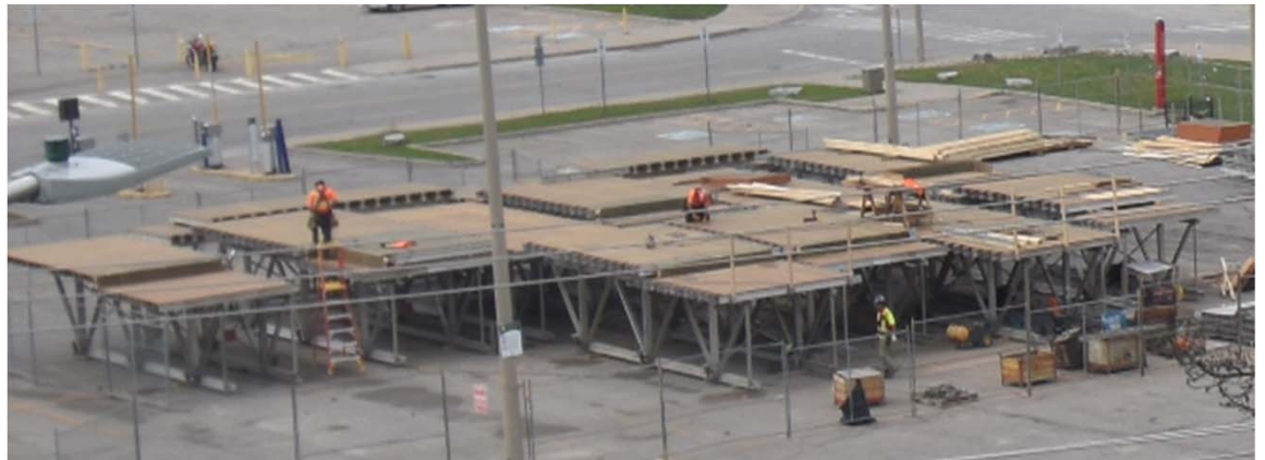
Formwork Assembly Yard at F2 parking
