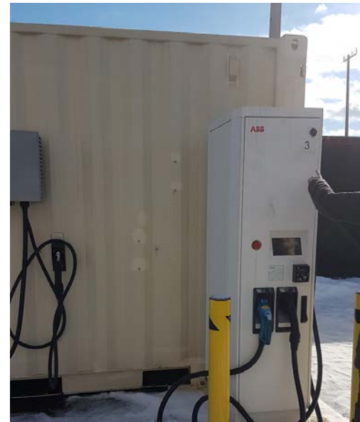
EV Charging Test Bed
