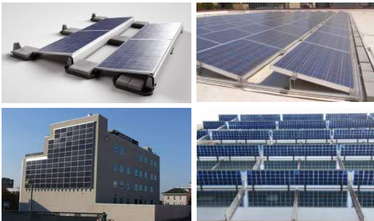
Figure 17. Examples for mounting of BIPV & BAPV
