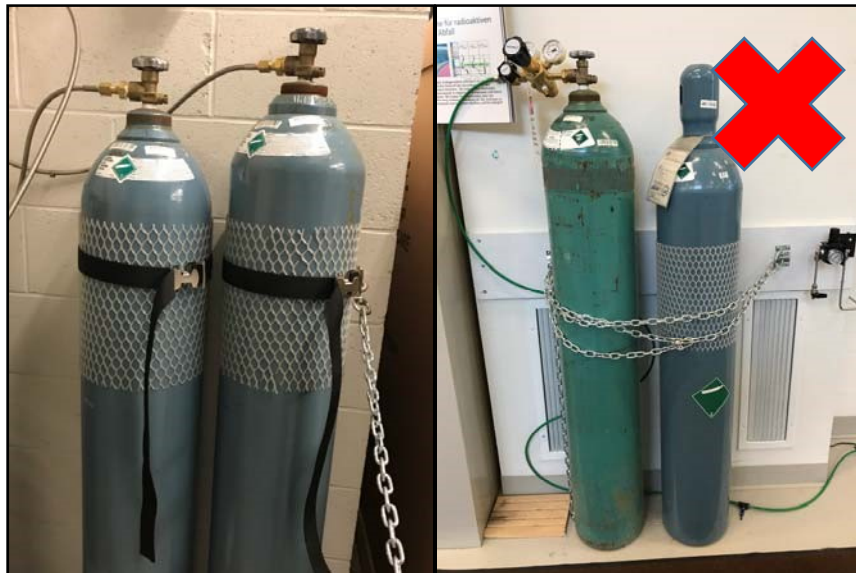
Figure 9 – Securing compressed gas cylinders.
