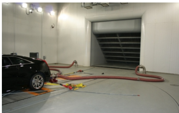
Dual closed-pipe vehicle exhaust extraction system
