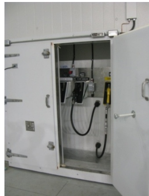
In-chamber refuelling station
