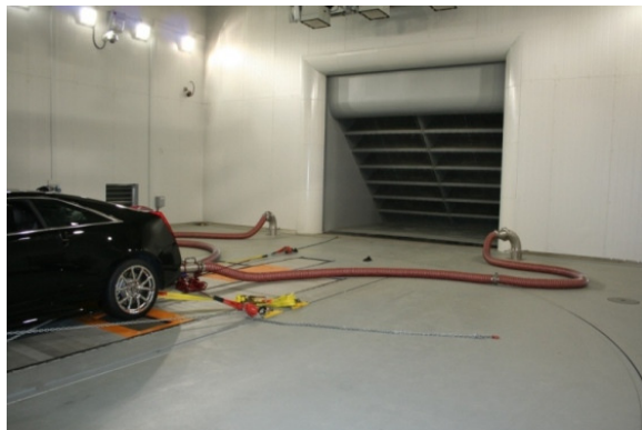
Dual closed-pipe vehicle exhaust extraction system
